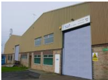
An outside view of the UK facility
